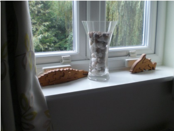
Figure 17. Window sensors monitoring the opening and closing of the windows in case study households.
