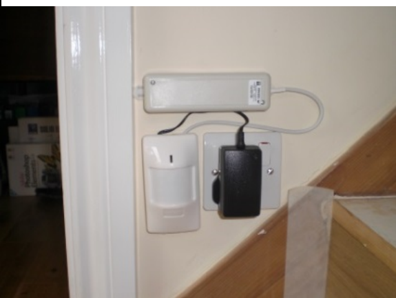
Figure 18. PIR sensors can monitor occupancy, but are very dependent on being placed in a suitable position.
