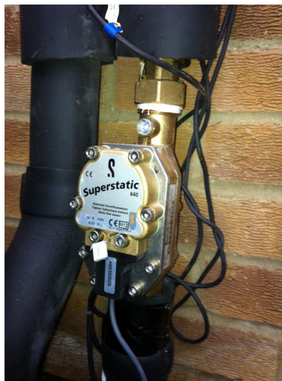
Figure 7. Heat flux meter installed in air source heat pump system to measure system heat output. Following installation, it should be fully insulated as per the piping around.
